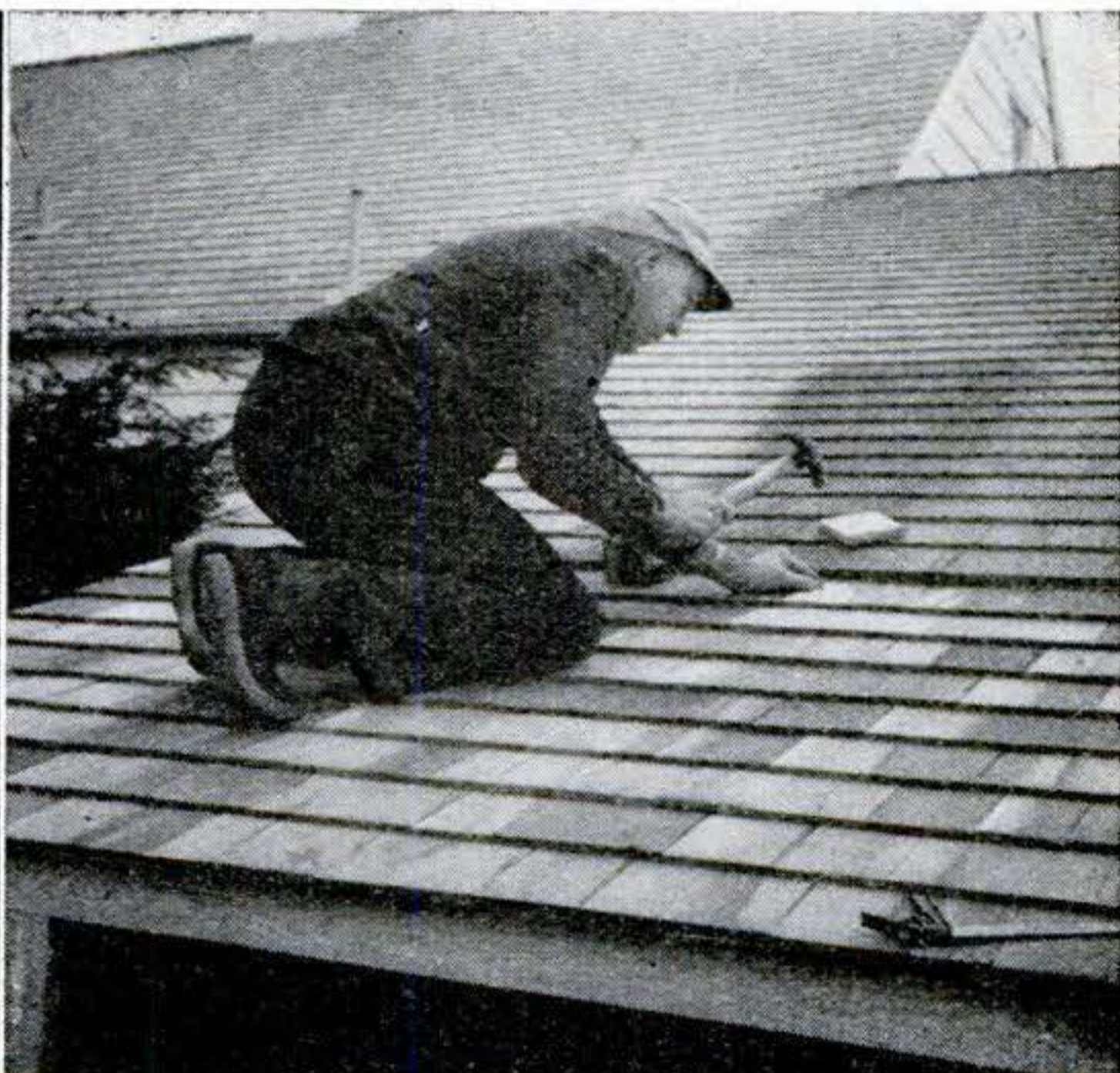
8 ROOF SHINGLES also match garage. Begin with double row at bottom and space courses evenly. Saw last two rows to fit tightly under eave. If fit is loose, install flashing.
